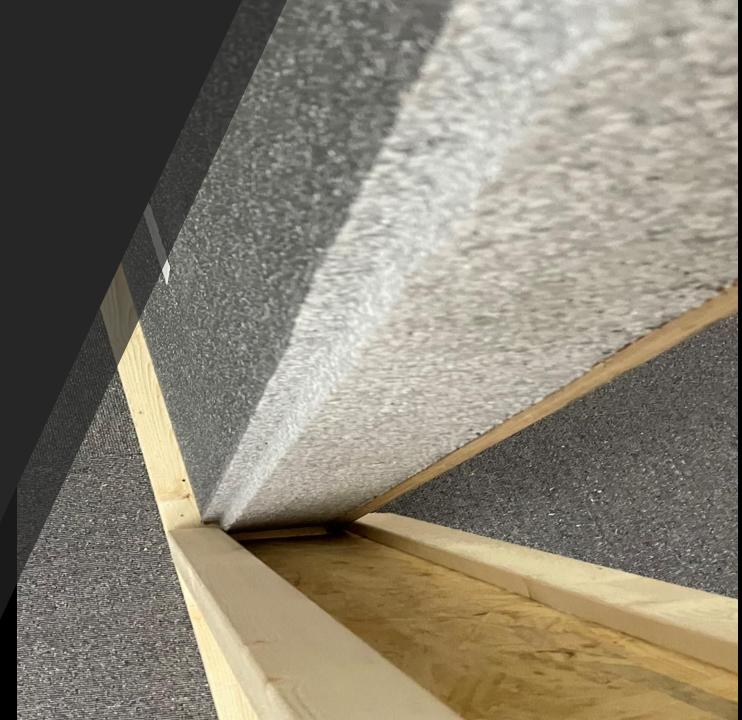
• Once panel is located fully into connector, check the panel and corner post are plumb.
